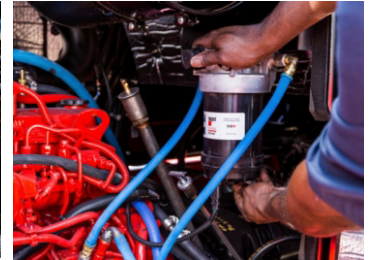
Easy Access to Fuel / Water Separator
